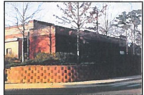
Do This: Refuse enclosures visible from public view will include hardscape materials that are the same as those
