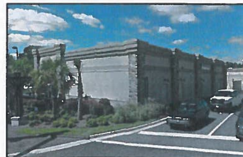
Don't Do This: A building that is positioned so that the rear is facing the main entry or gateway to the development. This approach is not inviting to pedestrians.
